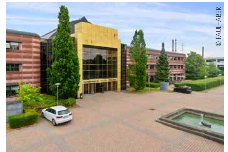
Das Scandinavian Trade Building von FAULHABER in Allerød, Gydevang 39-41.
